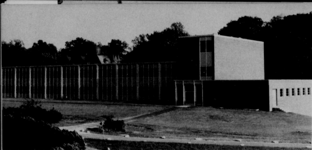
Wright Hall — New Science Building
